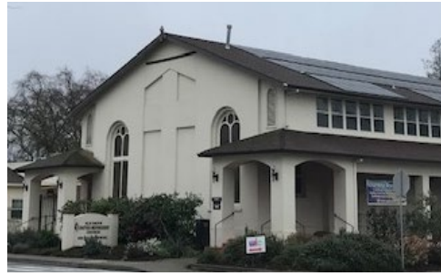
Elk Grove (Satellite) United Methodist Church 8986 Elk Grove Boulevard Elk Grove, CA 95624
